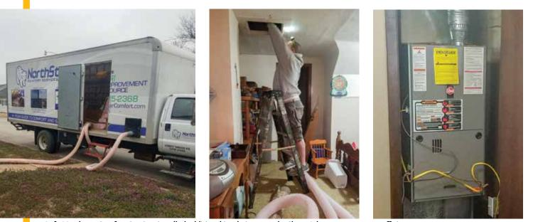
Left: Northstar Comfort Services installed additional insulation to make Sharon's home more energy efficient. Center: Northstar added 10.5 inches of insulation to Sharon's attic. Properly insulating a home is one of the simplest and most cost-effective ways to reduce energy use.
